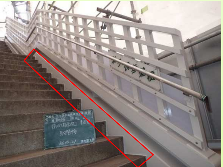
階段端部シーล材充填
