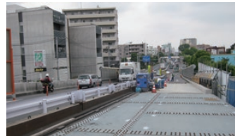
Replacement of bridge deck
