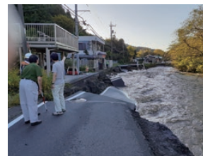
Damage caused by the disaster
