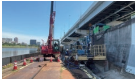
Seismic retrofitting of revetments (Sumida River)
