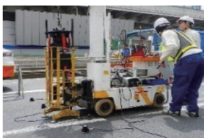
Taking measurements on an actual bridge (Weight-drop test)
