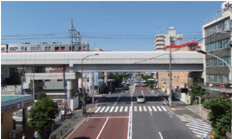
Keisei Oshiage Line (Oshiage-Yahiro Stations) continuous grade separation project
