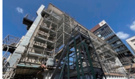
Seismic retrofitting of floodgates (Nihonbashi Floodgate)
