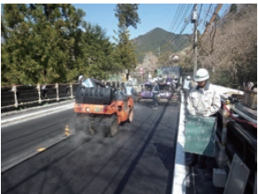
Repair of bridge deck surface
