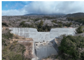
Sabo dam to protect houses from debris flows (Takigawasawa, Oshimamachi)
