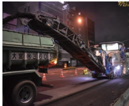
Road surface repair
