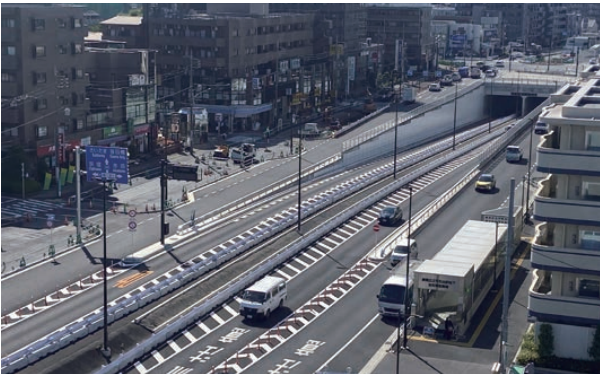
Radial Route No. 35 (Heiwadai Tunnel)
