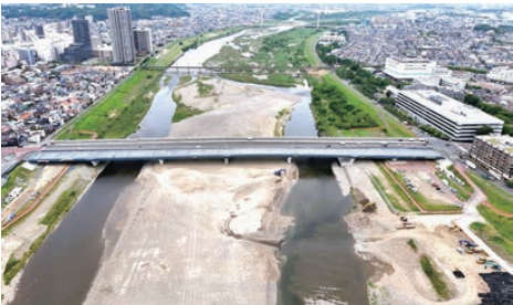
Sekido Bridge (under construction)
