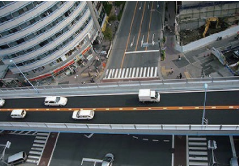
Shinkoiwa Overpass (Aerial view of the Tatsumibashi intersection)
