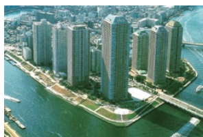
Super levee (Sumida River in the Okawabata district)
