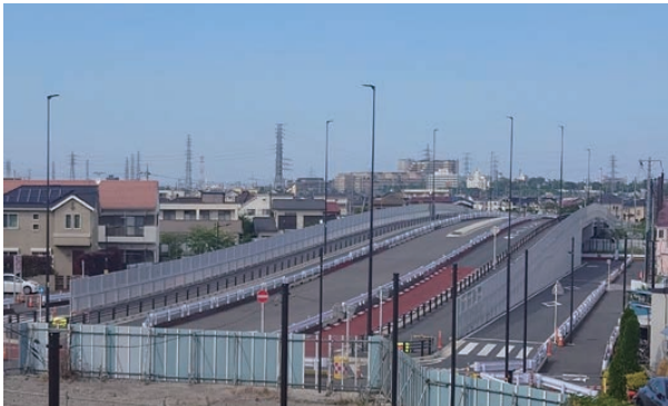
Fuchu Route No. 3-2-2 (2) (intersection with JR Nambu Line railroad)
