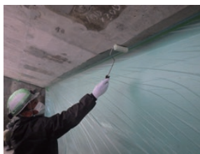
Repairs to concrete
