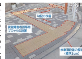
Barrier-free improvements on Waseda-dori Avenue (Shinjuku-ku)
