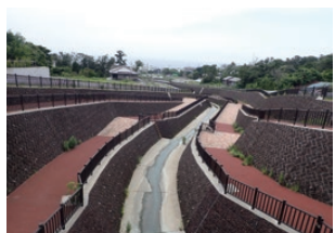
Okanasawa River channel works
