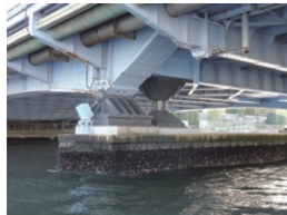
Reinforcement of bridge bearings
