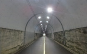
Enhancement of inner surface with reinforcing members
