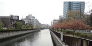
Earthquake-proof revetments (Oyokogawa River)
