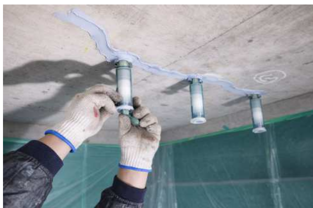
ひび割れ補修
