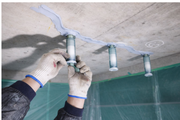
ひび割れ補修
