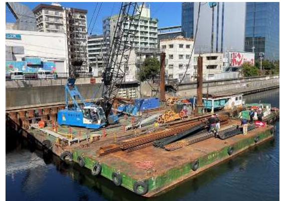
④既設矢板引抜
