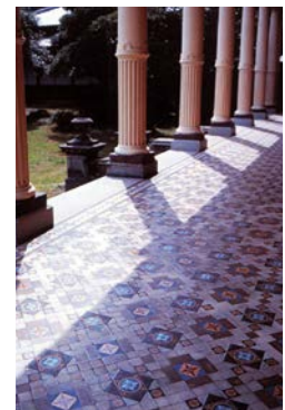
Tile laid on the first floor Veranda
